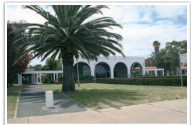
ABOVE: Balcatta Senior High School, Balcatta (1966-1969)
