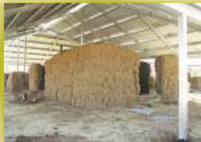
The Halls Creek Post Office ruins are now protected by a freestanding roof. Photo courtesy Derek Keene, Halls Creek.
