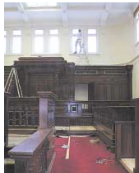
Works in progress in Courtroom Two.
