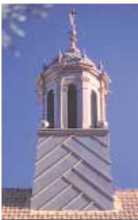
Reinstalled Cupola on the Methodist Ladies College Centenary Building.
