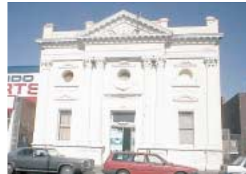
Victoria Hall prior to conservation works.
