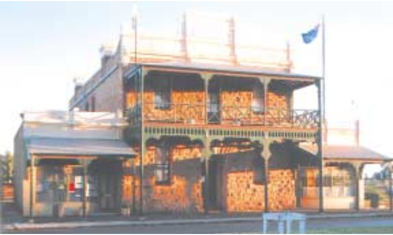
The Shire Offices is one of the few two storey buildings in Cue.
